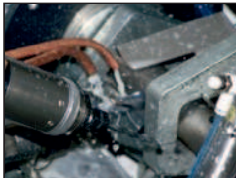
Photo of the drilling operation
